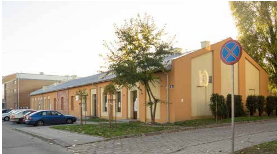
OŚRODEK KULTURY W ZABYTKOWEJ KANTYNIERZE | A COMMUNITY CULTURAL CENTRE IN THE HISTORICAL BUILDING OF A FORMER MESS-ROOM
